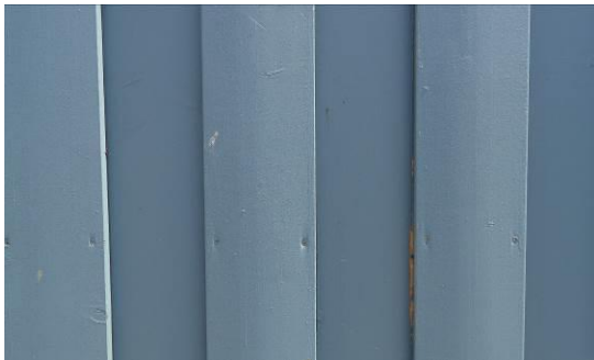
Boden-Deckel-Schalung
